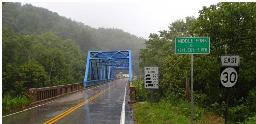
Aging steel truss structure over Middle Fork of Kentucky River
